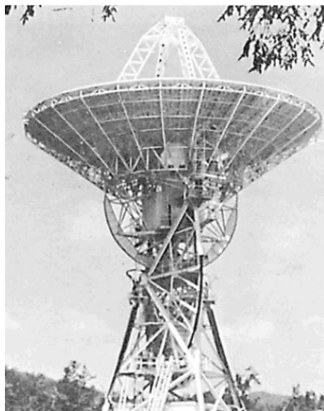
Figure 9: Example of an XY antenna mount showing the two large gears.
