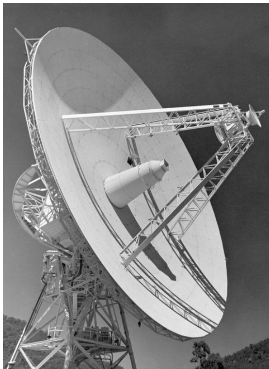
Figure 10: Showing the Antenna with Cassegrain feed system [Attribution]
